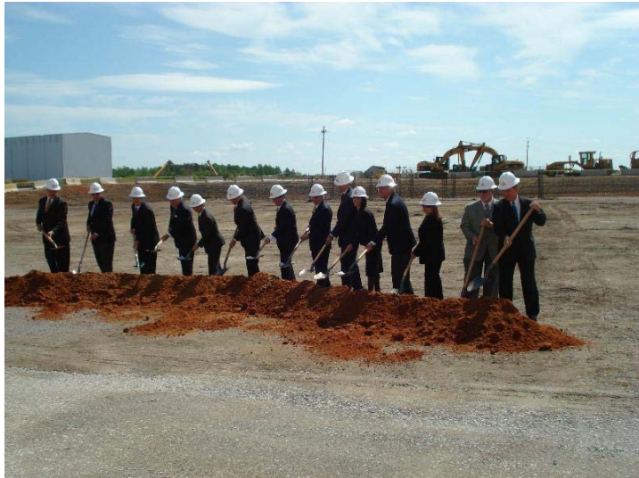
Groundbreaking Ceremony for CO 2 Capture Unit, Plant Barry (Bucks, AL)
