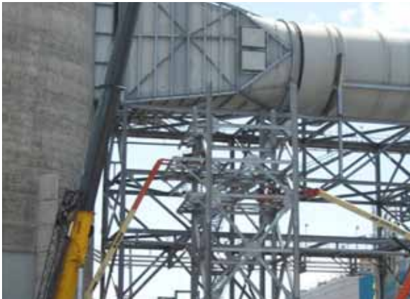
The 25 megawatt capture unit will tap into Barry Unit 5 post-scrubber. 3.5% of Unit 5's flue gas will be routed to the capture unit.
